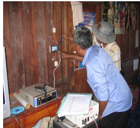
Checking of installation by PESCO
