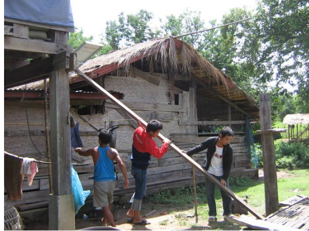
Setting up of a mast with solar panel
