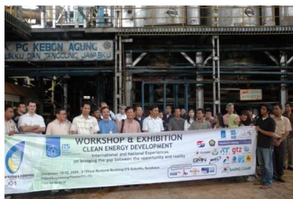
Figure 1: Biomass power plant
