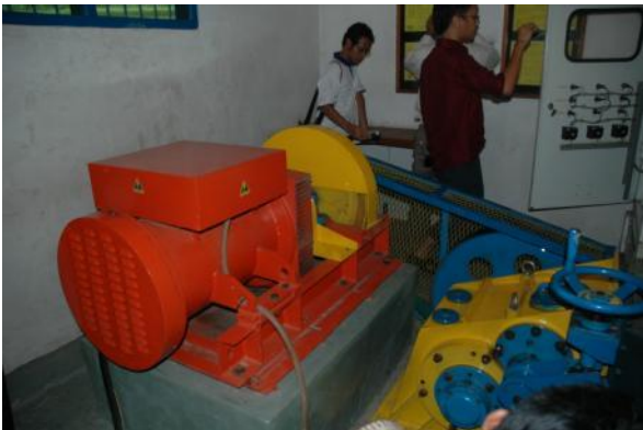
Figure 2: Micro hydro generator
