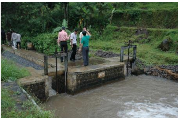
Figure 3: Micro hydro power plant
