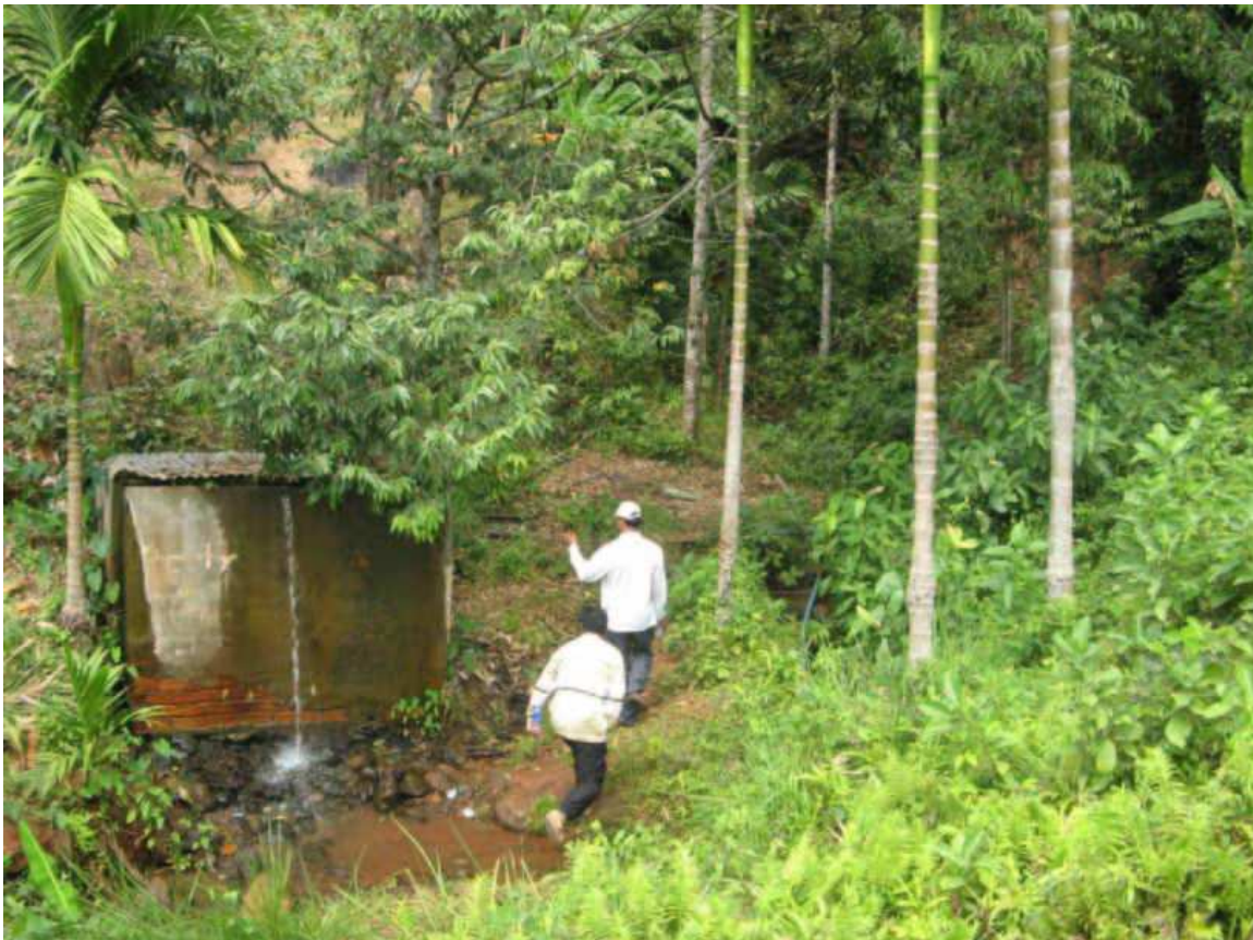
Figure 4 Collection tank for water supply – potential location for powerhouse
